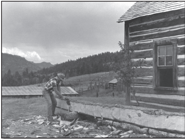
Figure 103—Hew down to the chalk line, removing the excess wood left after scoring.
